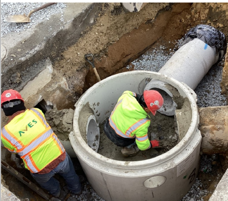
The Contractor will install new storm sewer pipes across West Street.
